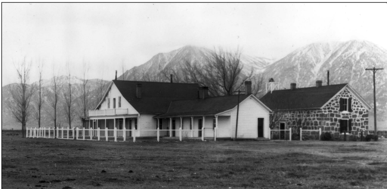
Dangberg Home Ranch, ca. 1910. Incorporated into the structure is the original cabin built by H. F. Dangberg in 1857.
